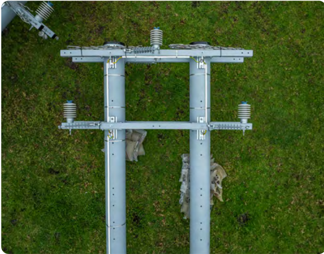
Figure 16 – Crossarm – to – Wagners CFT pole connections
