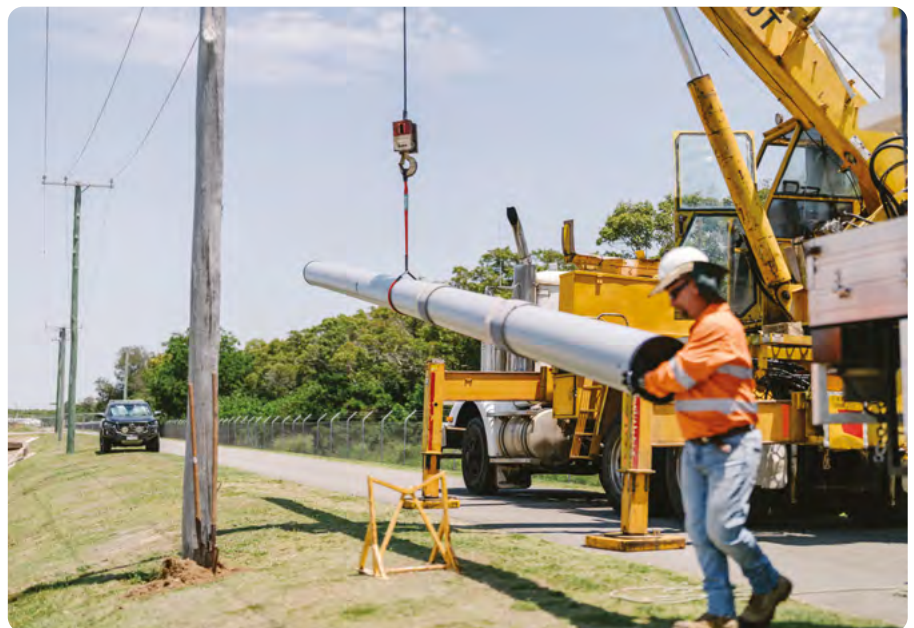
Figure 20 – Wagners CFT pole and crossarms are being installed into position
