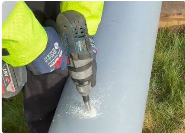
Figure 2 - Drilling on the pole
