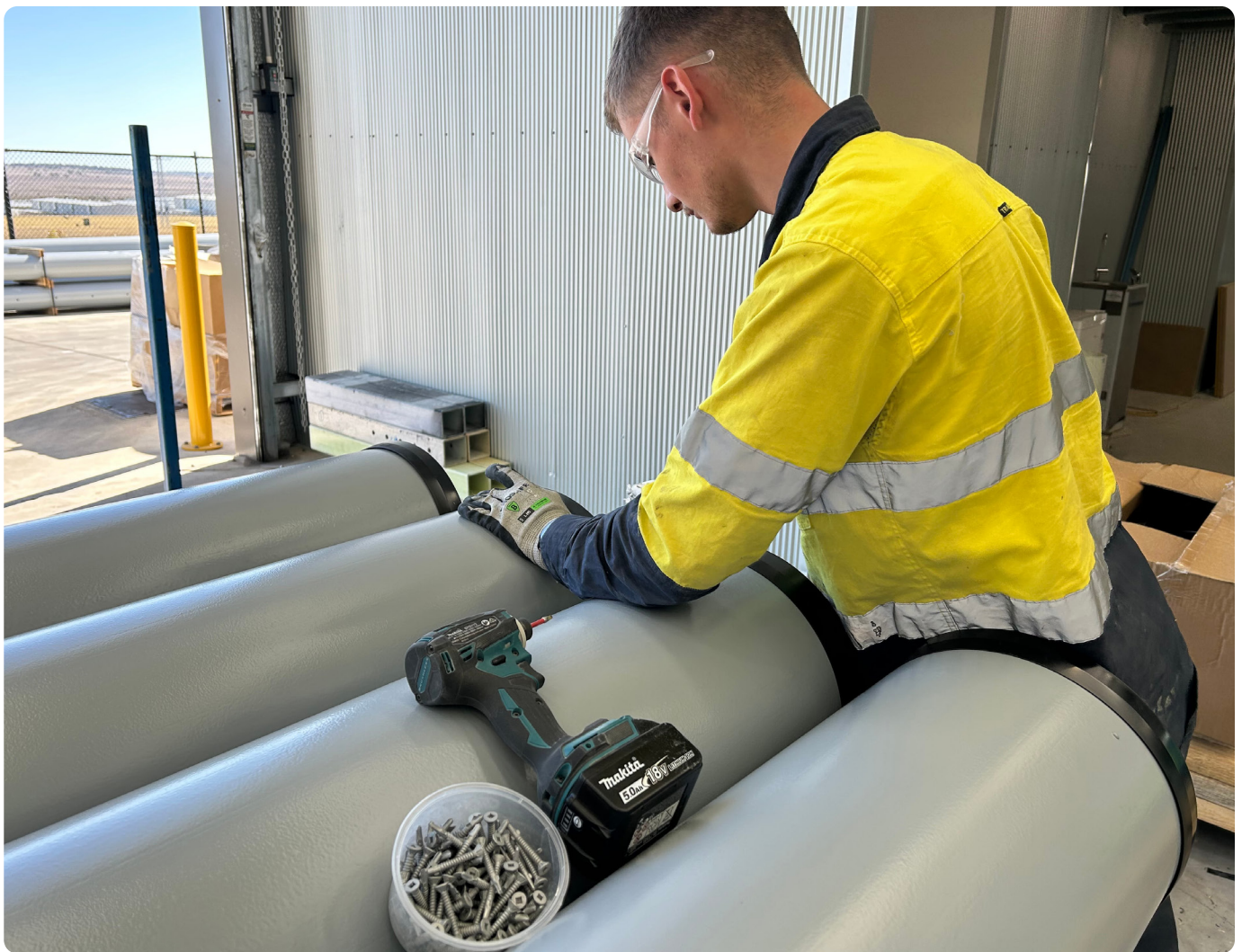
Figure 1 - Predrilled Wagners Pole
