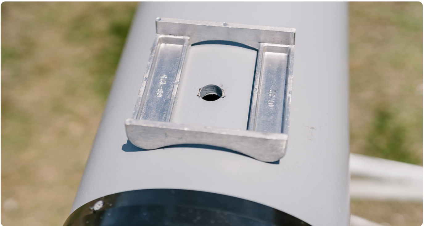
Figure 5 - Photo of the predrilled pole
