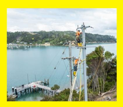
There's widespread belief that FRP utility poles are vulnerable to degradation in harsh outdoor environments, particularly under intense ultraviolet (UV) exposure or in coastal and marine regions. Because FRP is a composite material, some mistakenly believe it will fade, weaken or break down and bloom like untreated plastics or raw fiberglass over time. However, this myth doesn't hold up under scrutiny.
