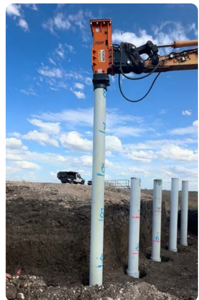
Impact/vibratory hammer
