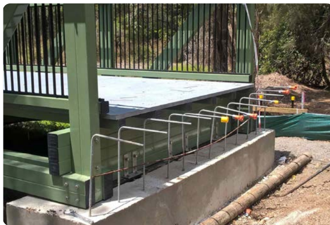
Landing of bridge structure on abutment
