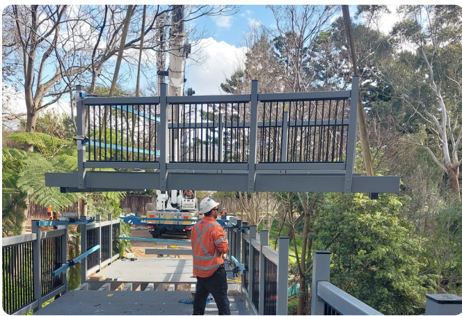
Lifting of partially assembled structures
