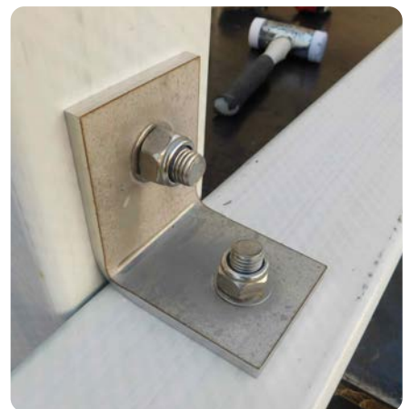
Threaded rods after installation leaving at least three threads past outer nut
