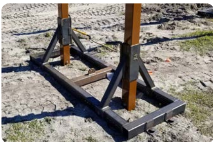
Positioning of piles using jigs
