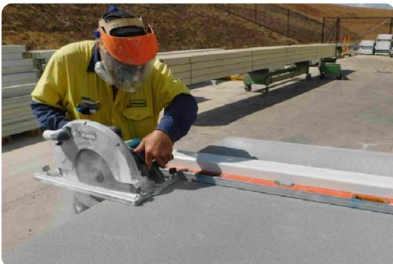
Cutting of decking using circular saw
