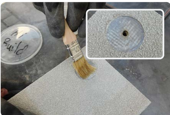
Sealing of holes in decking
