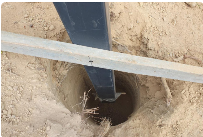
Post with insert and rod at the bottom
