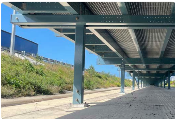
Post fixed to concrete using bolted shoe bracket and chemset anchor connection
