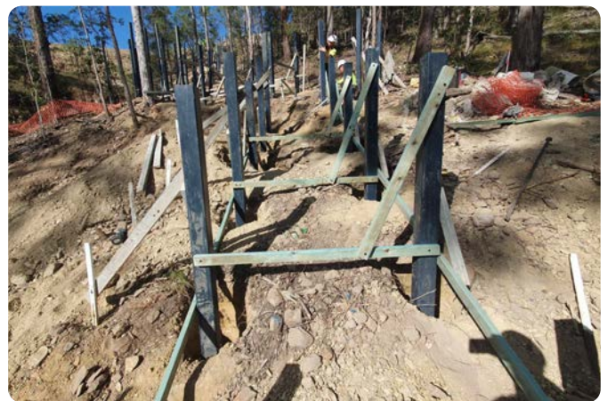
Bracing and aligning of the post for bored pier
