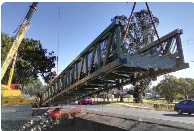
Lifting of pre-assembled bridge members
