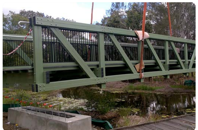
Lifting of pre-assembled bridge members
