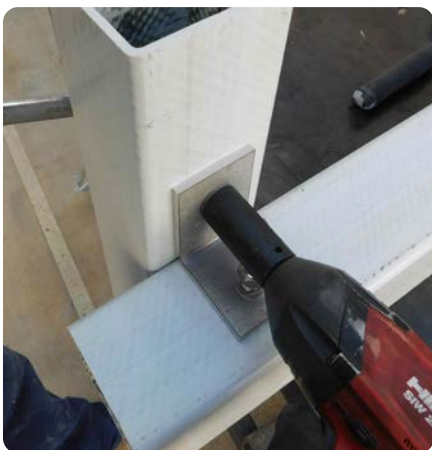
Tightening of nyloc nut using impact wrench
