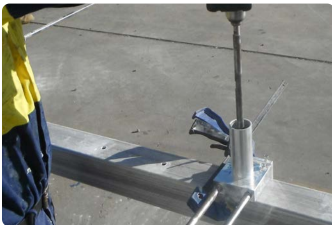
Drilling of composite member
