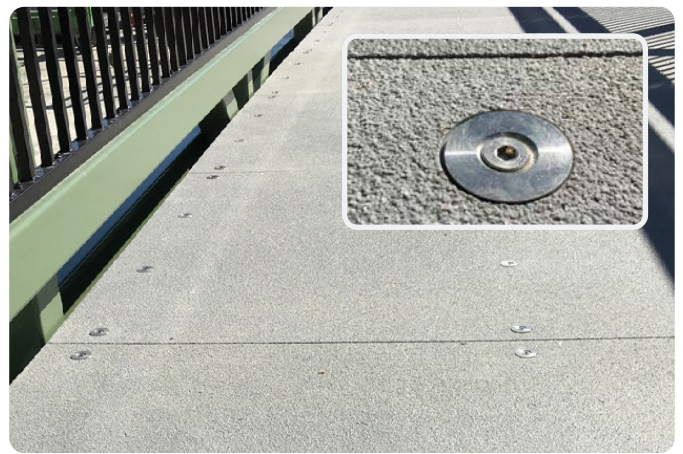
Fixing of deck using countersunk/oversize washer
