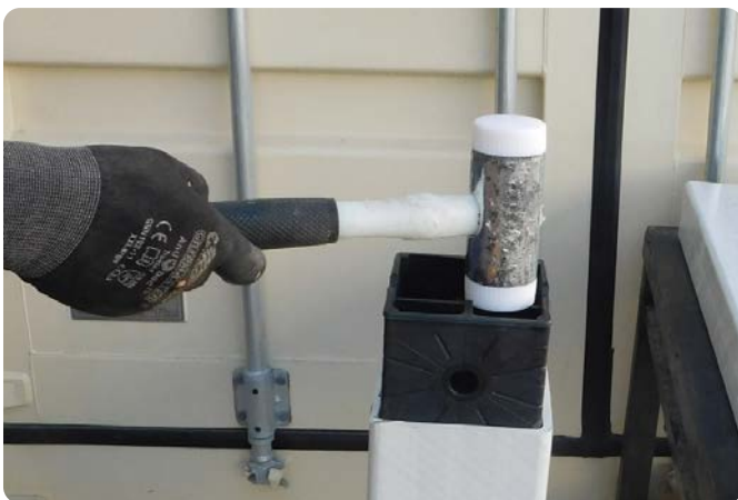
Hammering of insert
