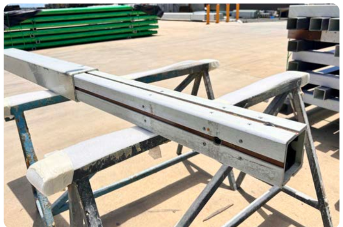
Pile splice fixed into a pile
