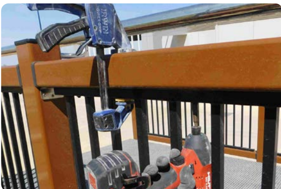
Clamping of balustrade and driving the screws
