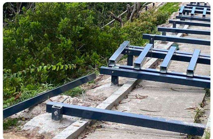
Post after concrete is poured
