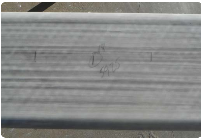
Marking of hole position before drilling
