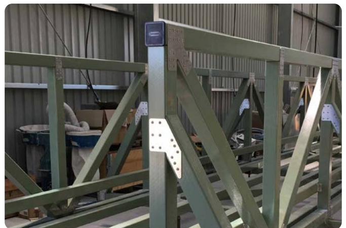
Riveted truss brackets vertical-outrigger
