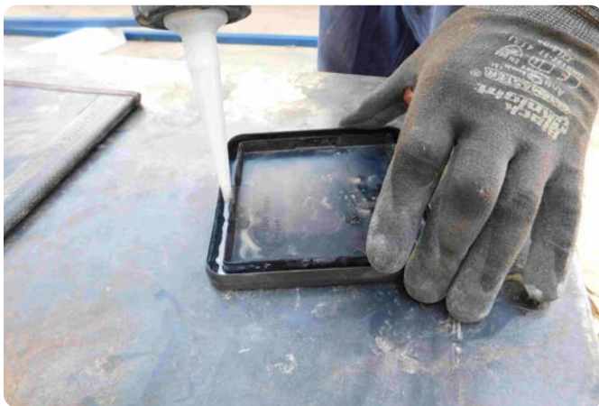
Adding Sikaflex in the groove of endcap
