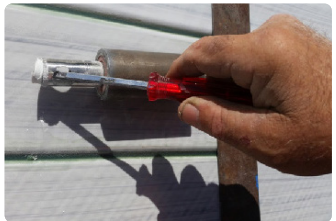
Pushing of slugs out after drilling
