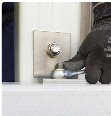
Tightening of nut using spanners
